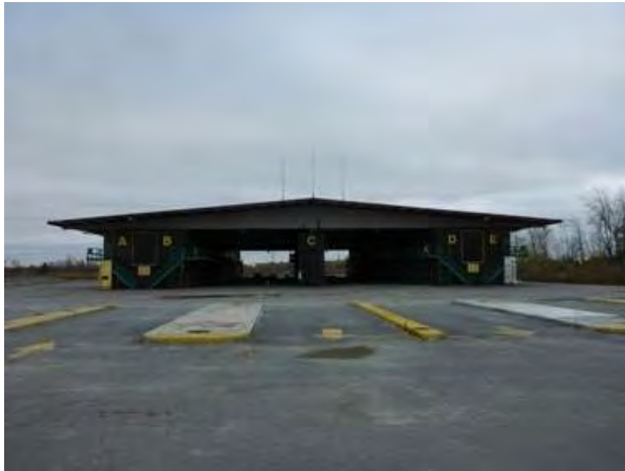
Image 5: Central loading station/mill looking south.
