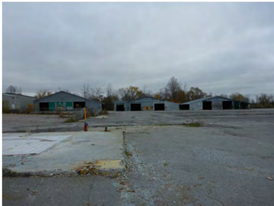
Image 4: A series of storage/warehouse buildings located south of the main Builder's Warehouse along the eastern property border. Photo taken looking east.
