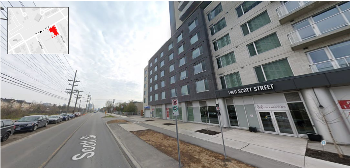
Figure 6.0 - Existing Site Conditions, View East Along Scott Street
