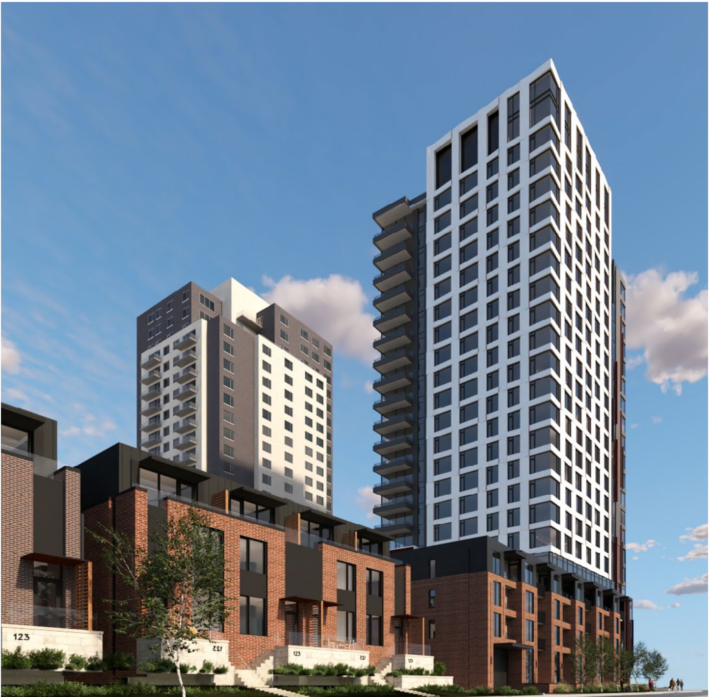
Figure 16.0 - View looking North along Clifton Road.
