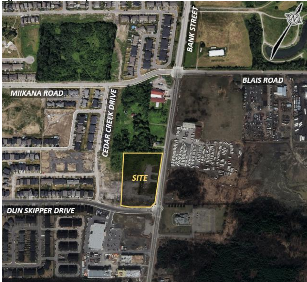
Figure 1: View of the Subject Site
