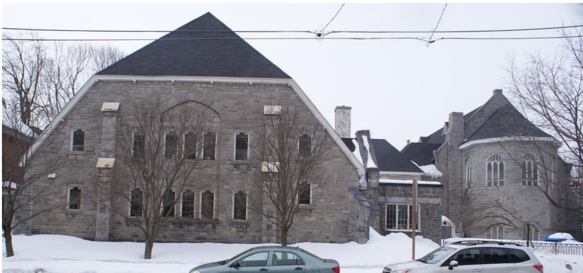
Figure 10: View of the Blackburn Avenue frontage with the 1934 Bate Memorial Hall (left) and the apse of the former All Saints Anglican Church (right). The plan calls for the demolition of Bate Hall. Source: Commonwealth 2023.
