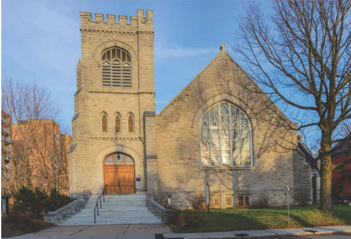
Figure 9: View of the main façade of the former All Saints Anglican Church, fronting onto Chapel Street. 2017.
