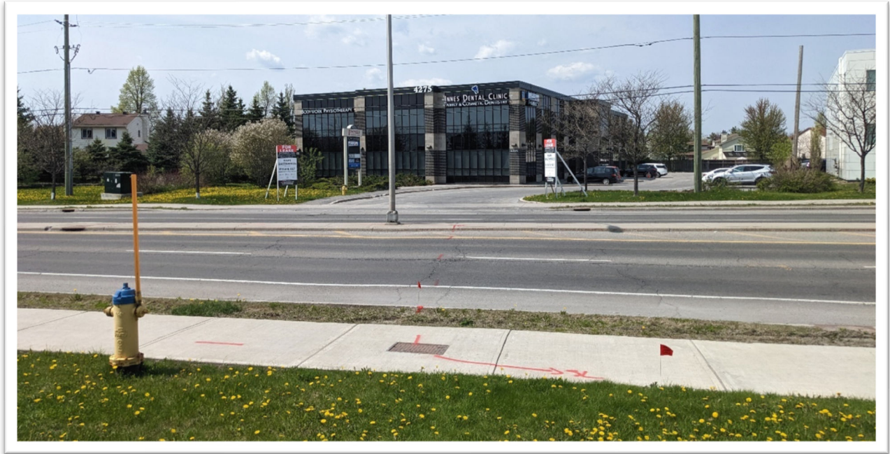
Photo 5: 4275 Innes Road, located 45 meters north of the Site.
