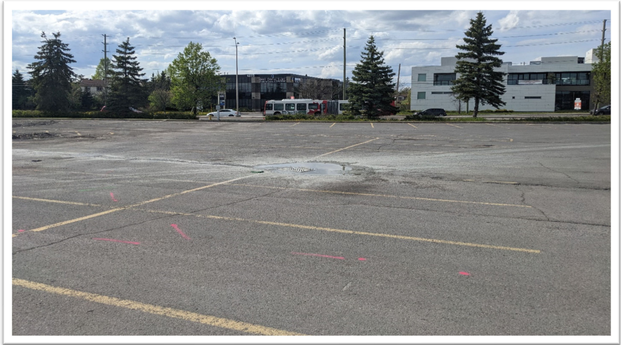
Photo 3: The eastern boundary of the Site, facing north towards Innes Road.
