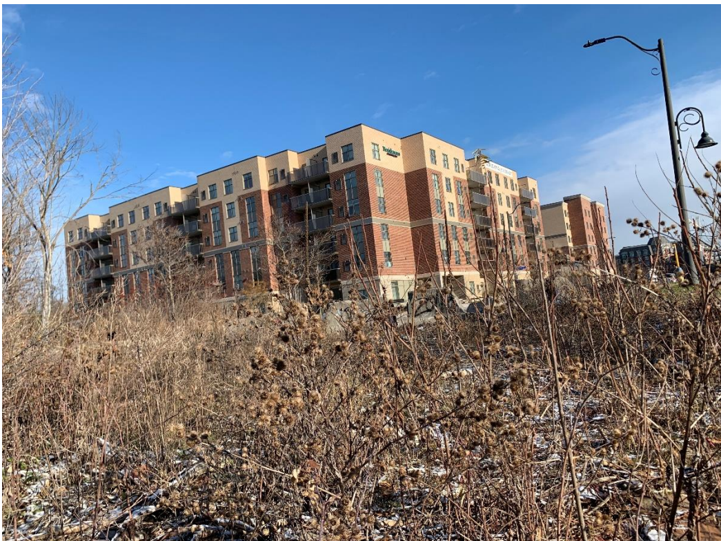
Photo 8: Commercial property located northeast of the Site.
