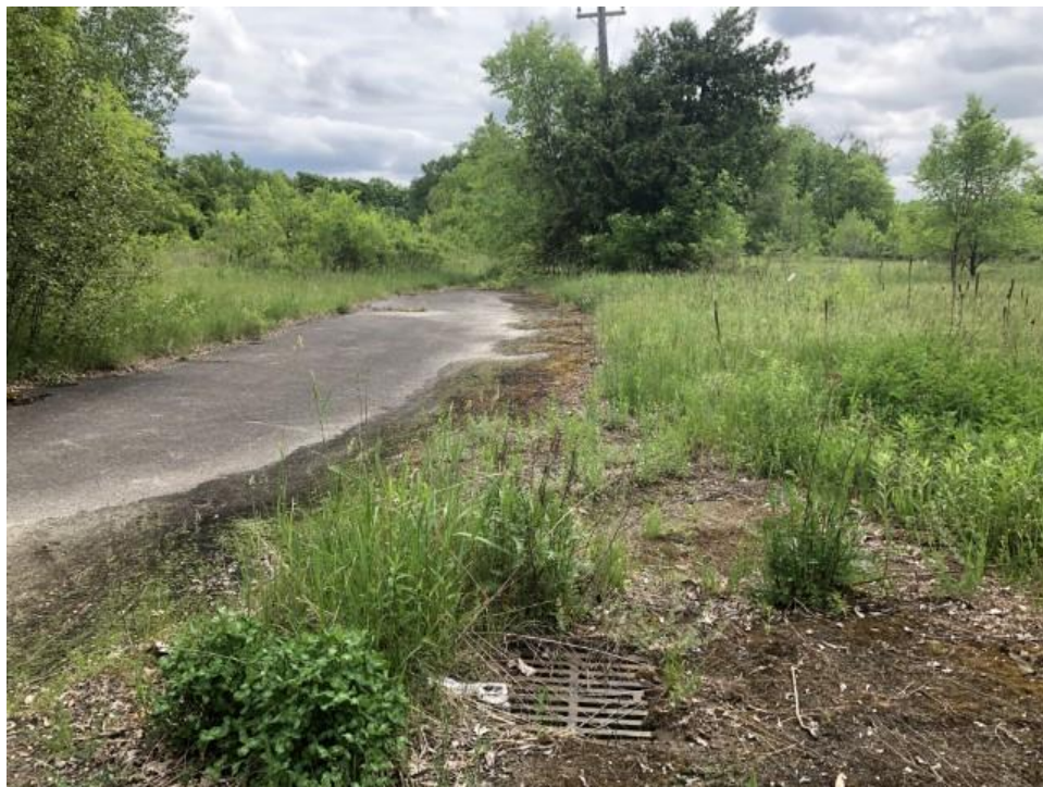
Photo 4: Typical off-site area to NE of Site showing former base infrastructure
