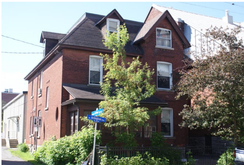
Figure 11: View of the 1902 Parsonage. The building is a brick-clad wood frame structure set on a coursed limestone foundation enclosed with a hip roof with a projecting bay enclosed with a gable roof. Source: Commonwealth 2024
