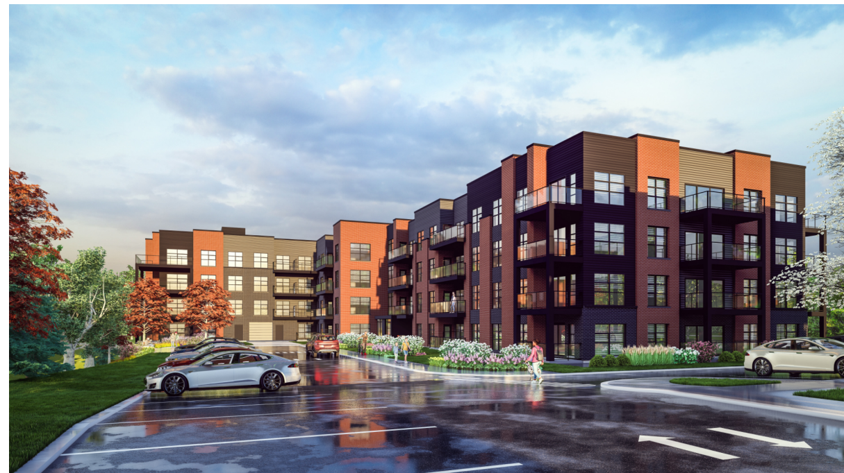
Figure 13.3 – Looking northeast towards Building C from internal visitor parking area (September 2024).
