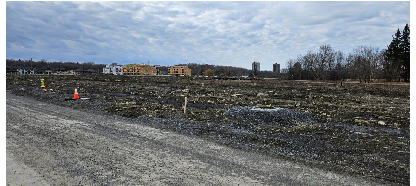
Figure 4.0 – View along Oshedinaa Street, looking southwest along Block 6 east property line (March 2024).
