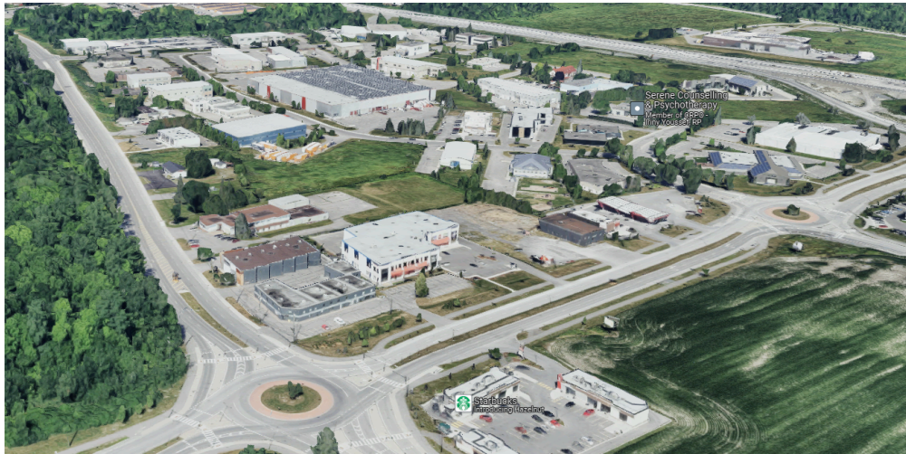
Figure 1: 1-2 storey buildings further west down Old Montreal Rd
