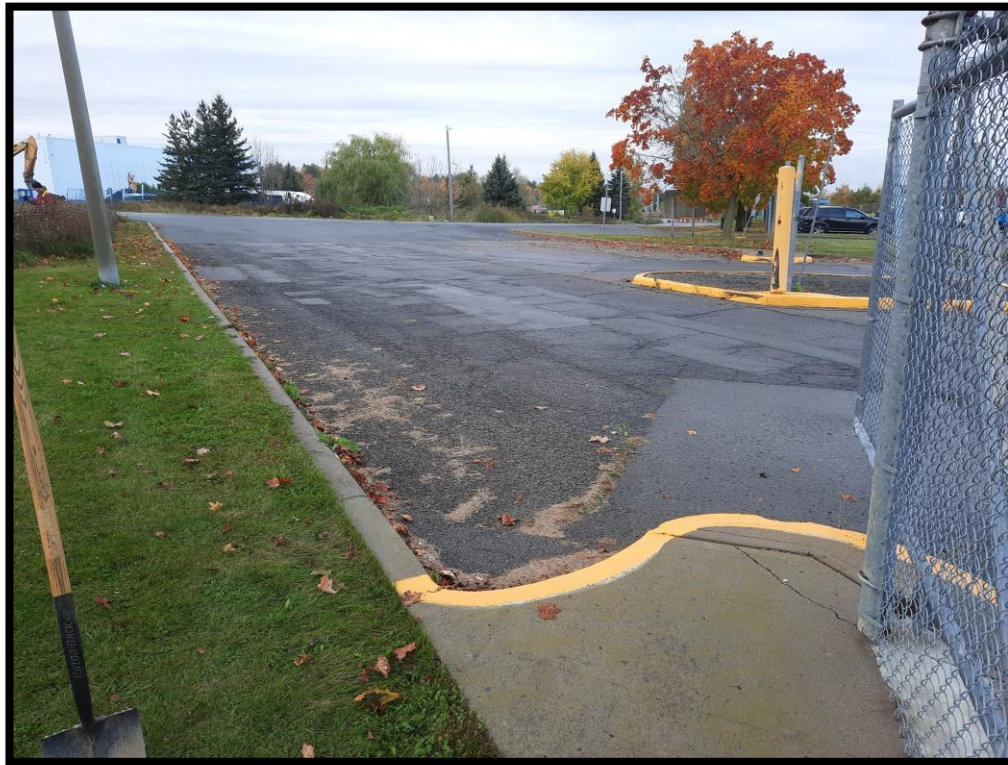
Figure 1: Dairy Drive along northwestern boundary (D002).
