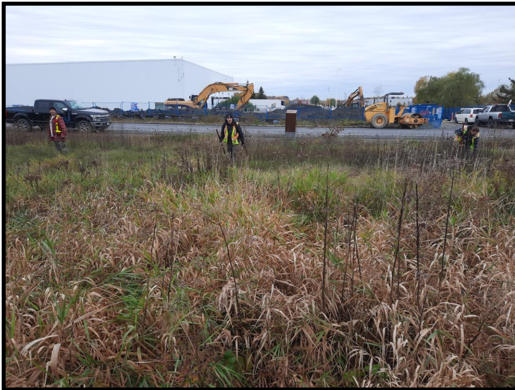
Figure 24: Test pitting in progress (D019).
