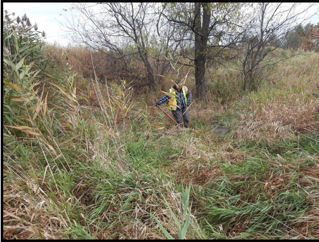
Figure 27: Test pitting in progress (D033).
