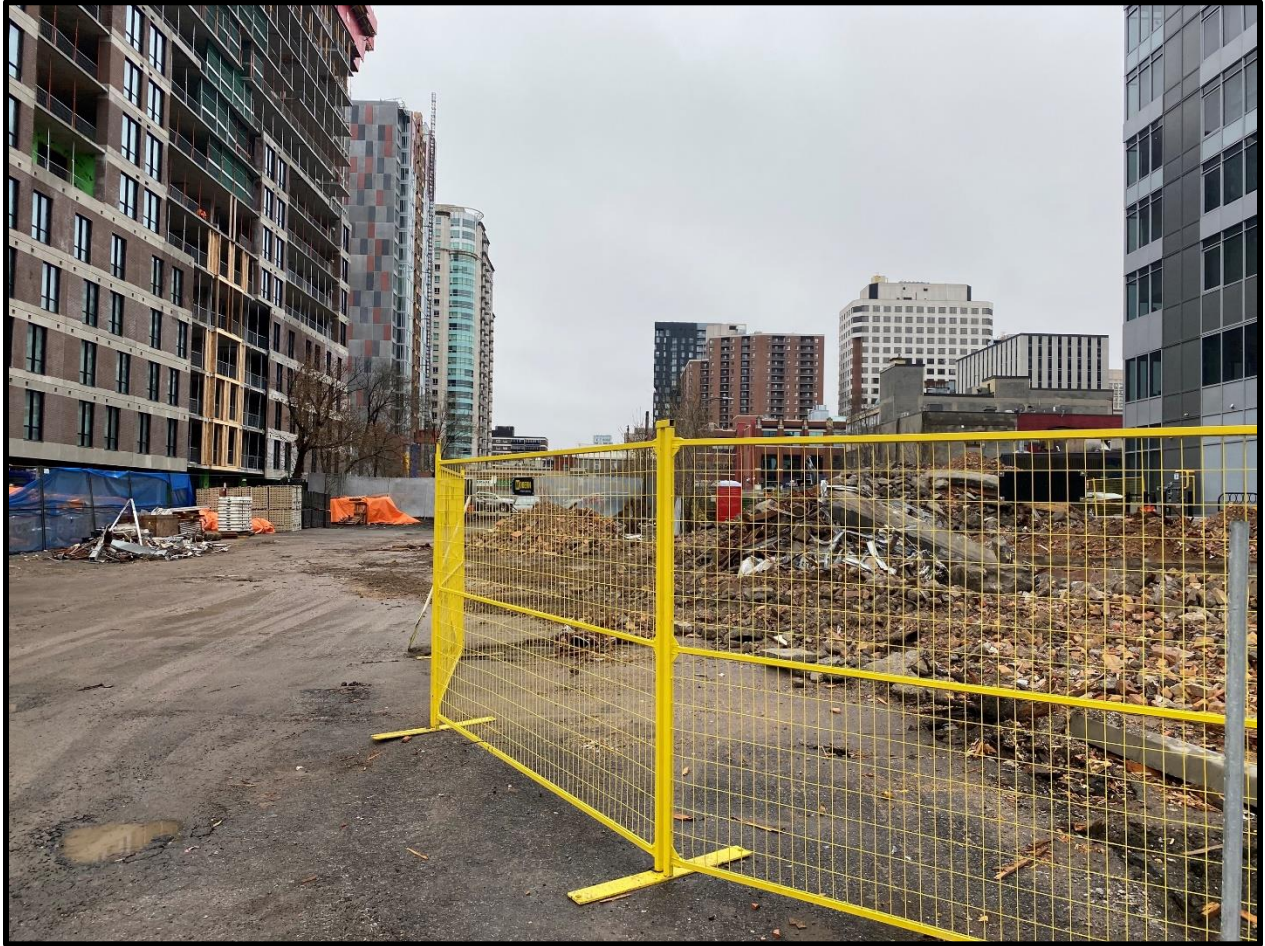
Photograph 3: View of demolished building (110 York Street), facing south.
