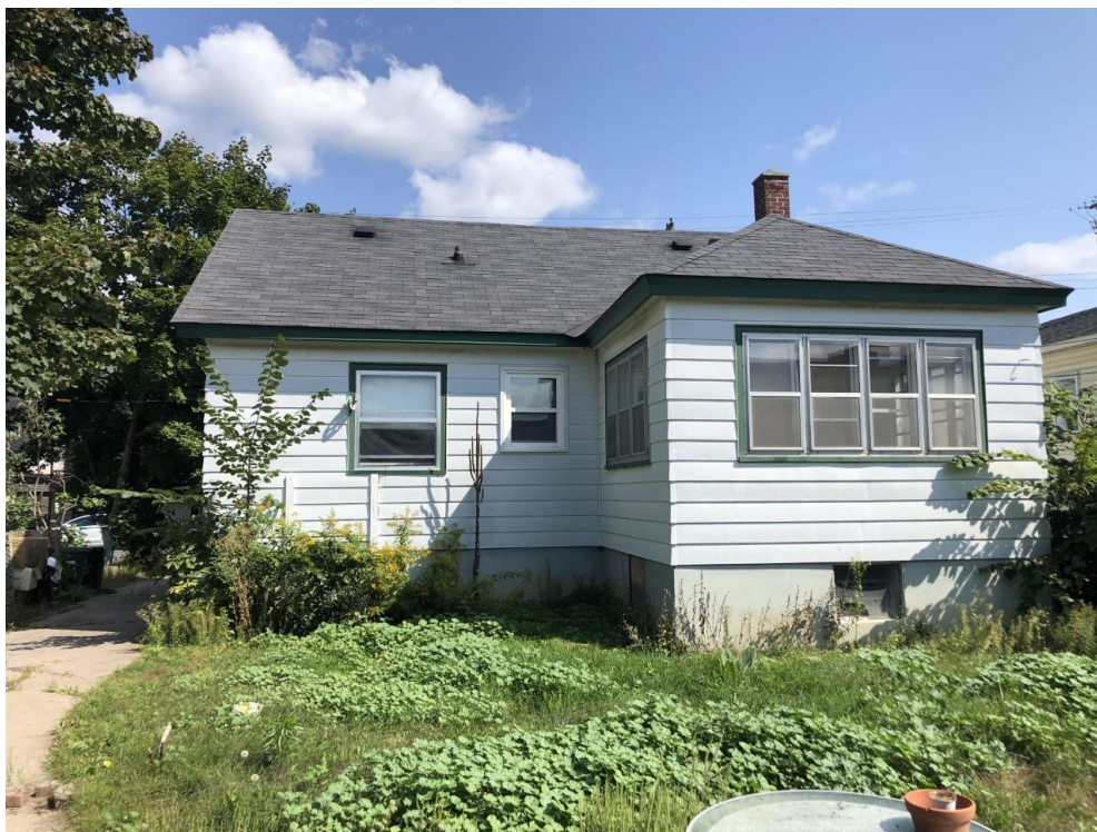
Photograph 2: View of the back of the residential dwelling, facing east.
