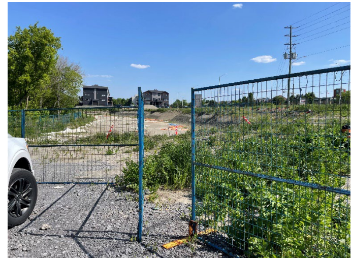
Looking south at the break in the fencing at the access road along Klondike Road
