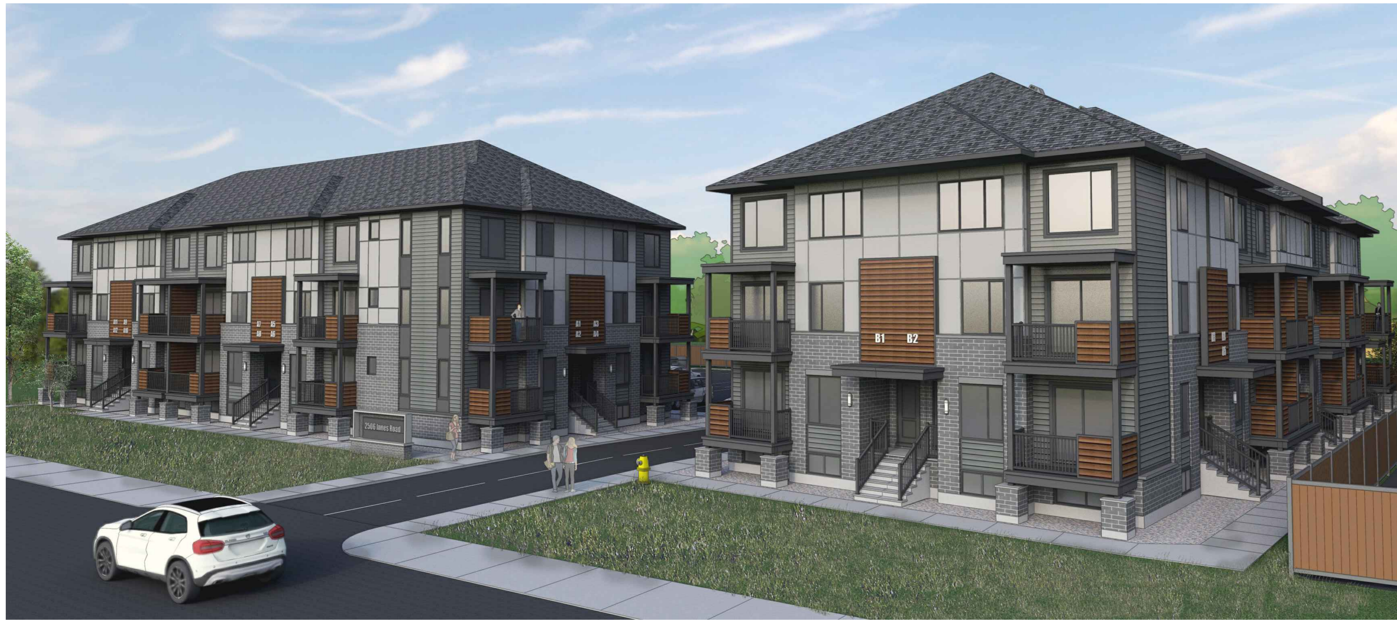
01 | VIEW ALONG INNES ROAD
