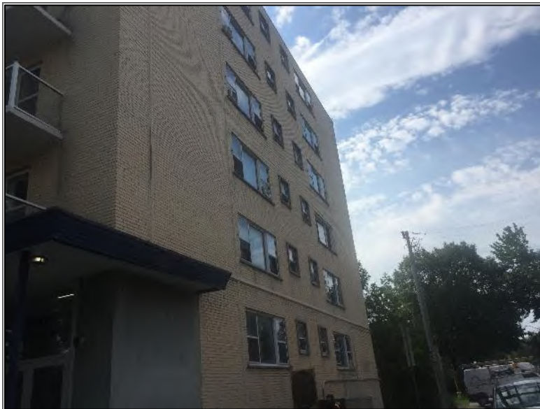
Photo 4 – Site Building (west elevation).
