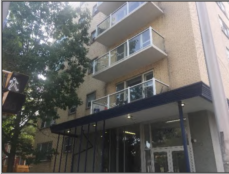
Photo 1 – Site Building (north elevation).
