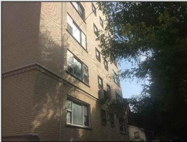
Photo 2 – Site Building (south elevation).
