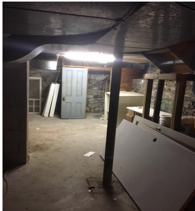
Photo 6: Typical Photo of unfinished stone foundation basement (2020 Site Visit).
