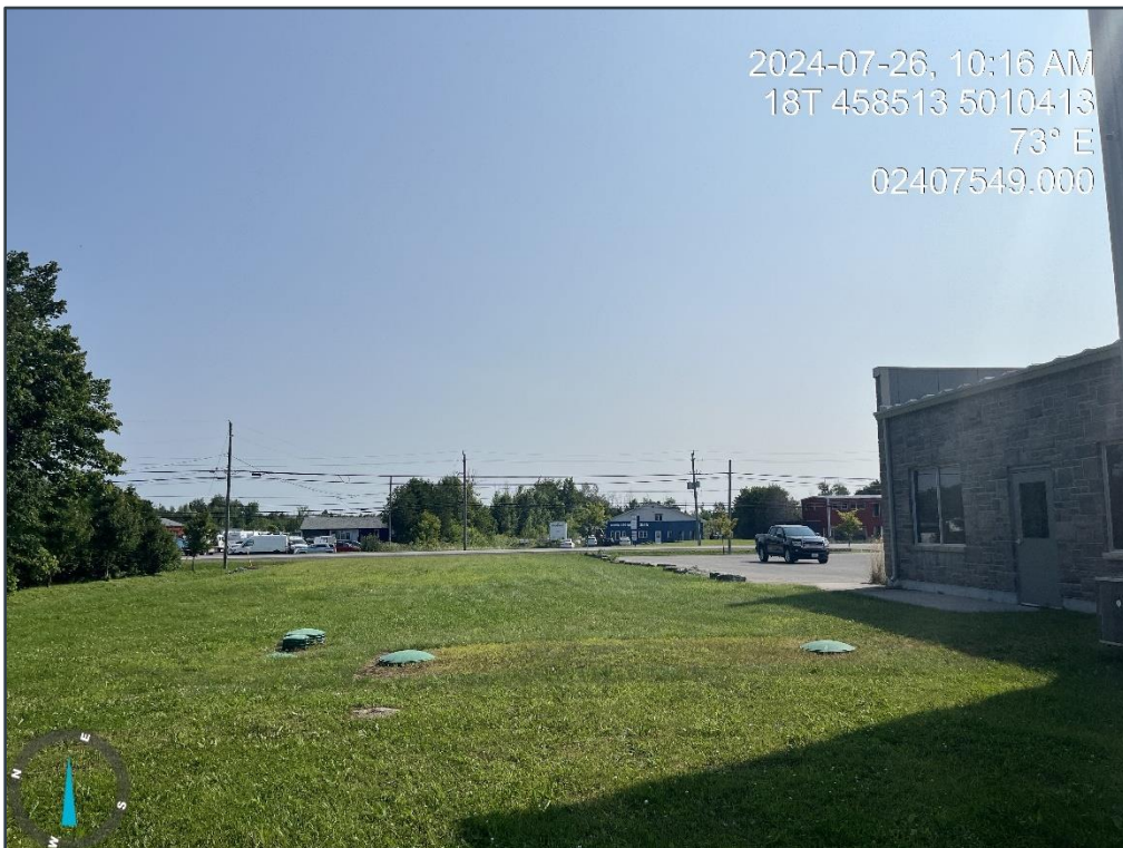
Photograph 10: Septic Tank Area (6622 Bank Street).
