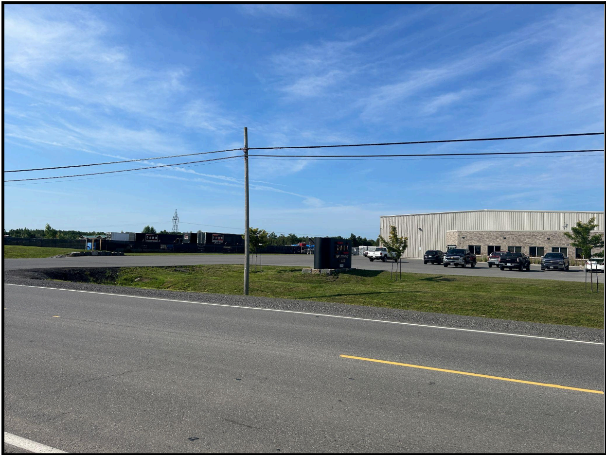
2. Front view of the existing building at 6622 Bank and the associated office space.
