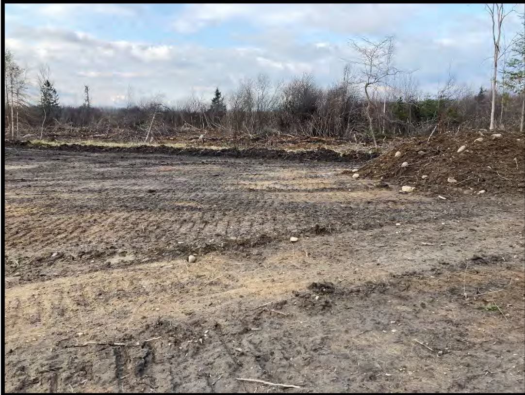
Figure 12: View of stockpiled stripped soil, exposing subsoil, and bulldozer tracks. (MH1174-D053)
