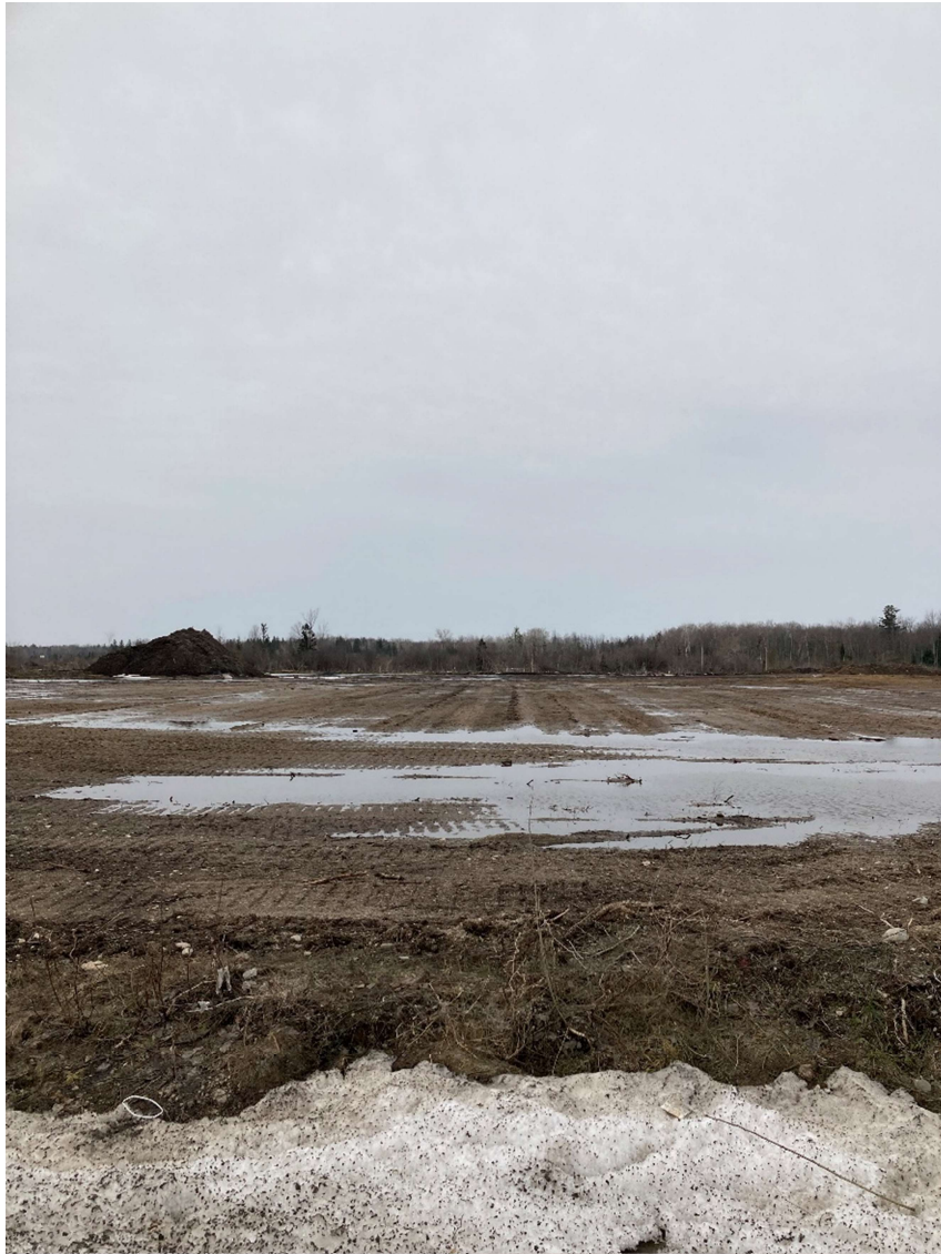
Photograph 3: Overview of 151 Wescar Lane (looking southwest)
