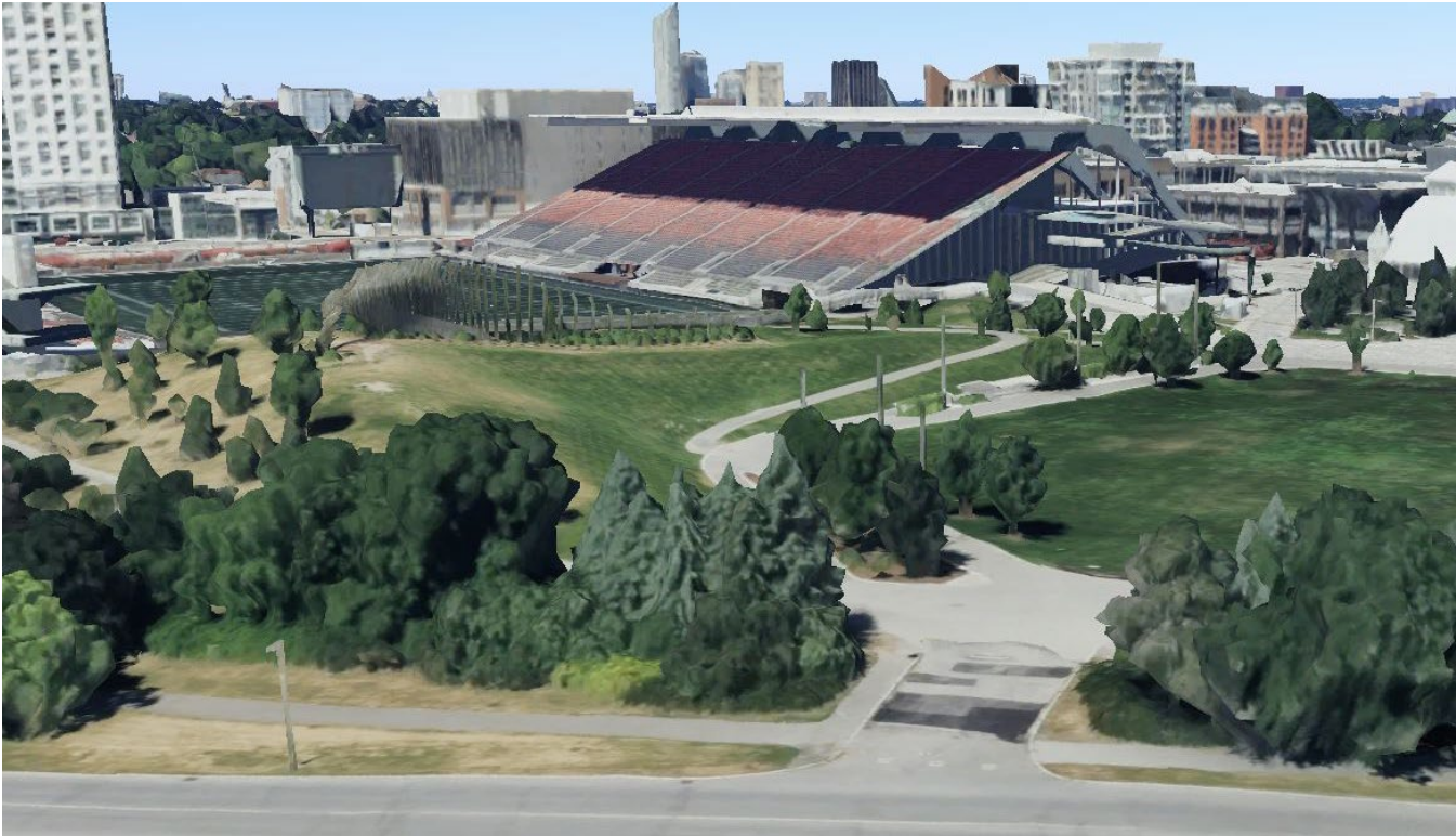
Figure 5. Existing Condition looking north-west.
