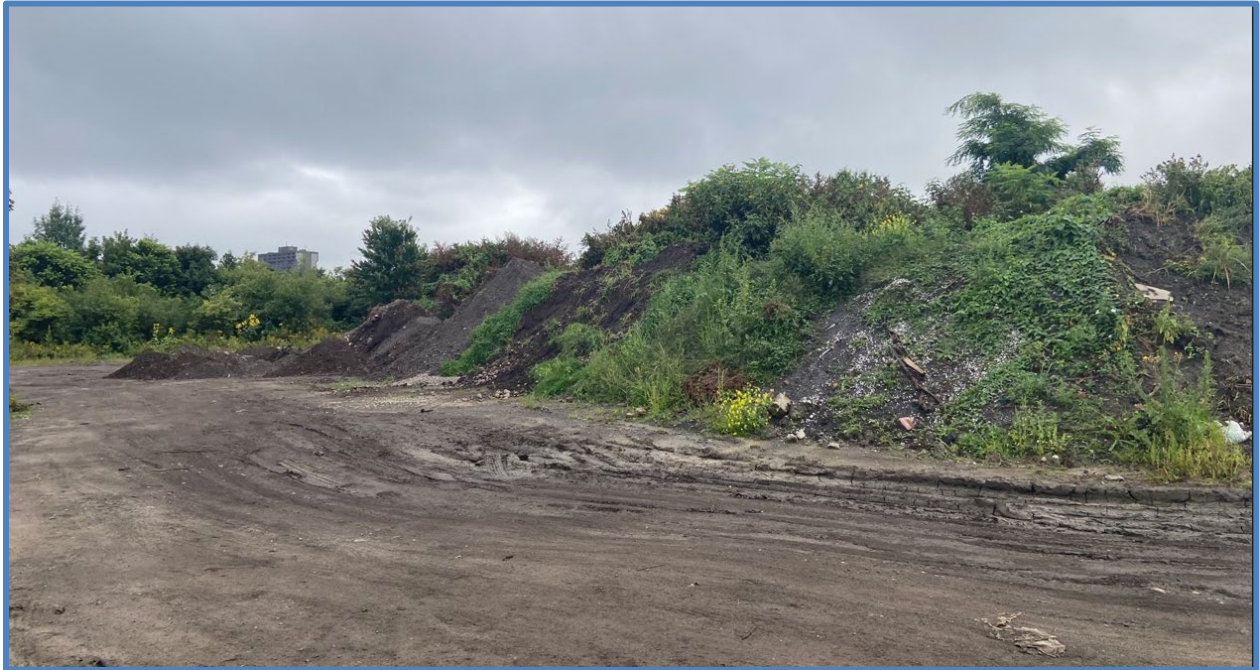
Figure 9: Unconsolidated Fill Piles.
