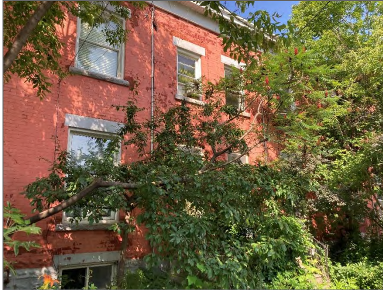
Photo 3 – Site Building A (east elevation).
