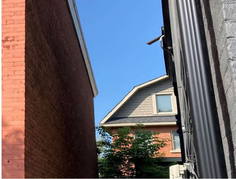
Photo 1 – Site Building A (north elevation).
