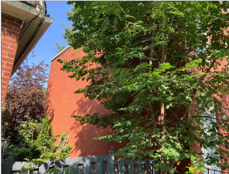
Photo 2 – Site Building B (south elevation).
