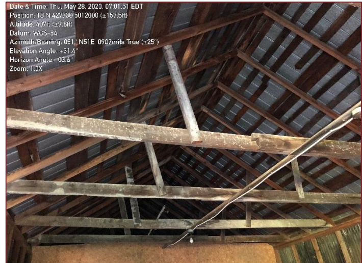
Site Photograph 4 – Inside Roof of Barn Structure
