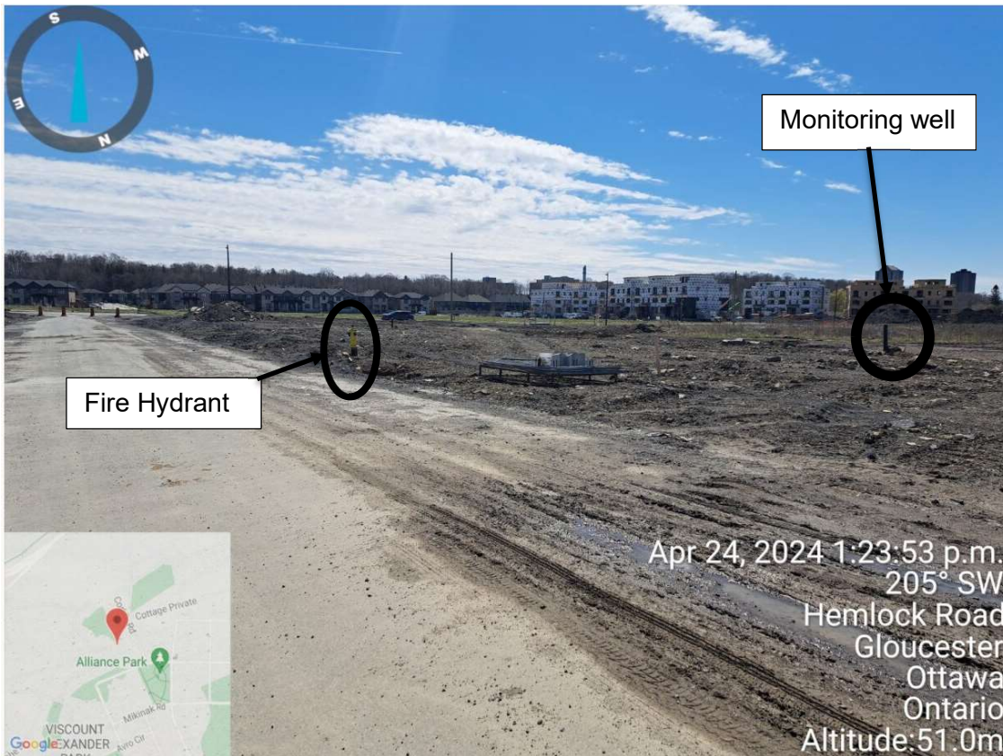
Standing at northeast side of Oshedinaa St. and looking towards southwest of Block 6 and Block 5 : No indications of existing slope greater or equal to 2 m in height or any settlement. Presence of service lines, monitoring wells, etc.
