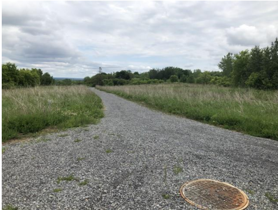
Photo 3: Northern portion of Site looking along sewer line
