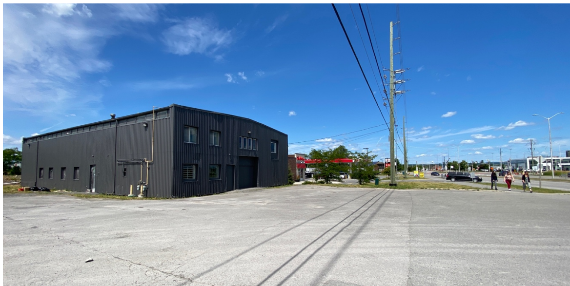
Figure 6: View of the site from the frontage of the property looking north along Trim Road. The black building on the left side of the photo is location on the subject property.
