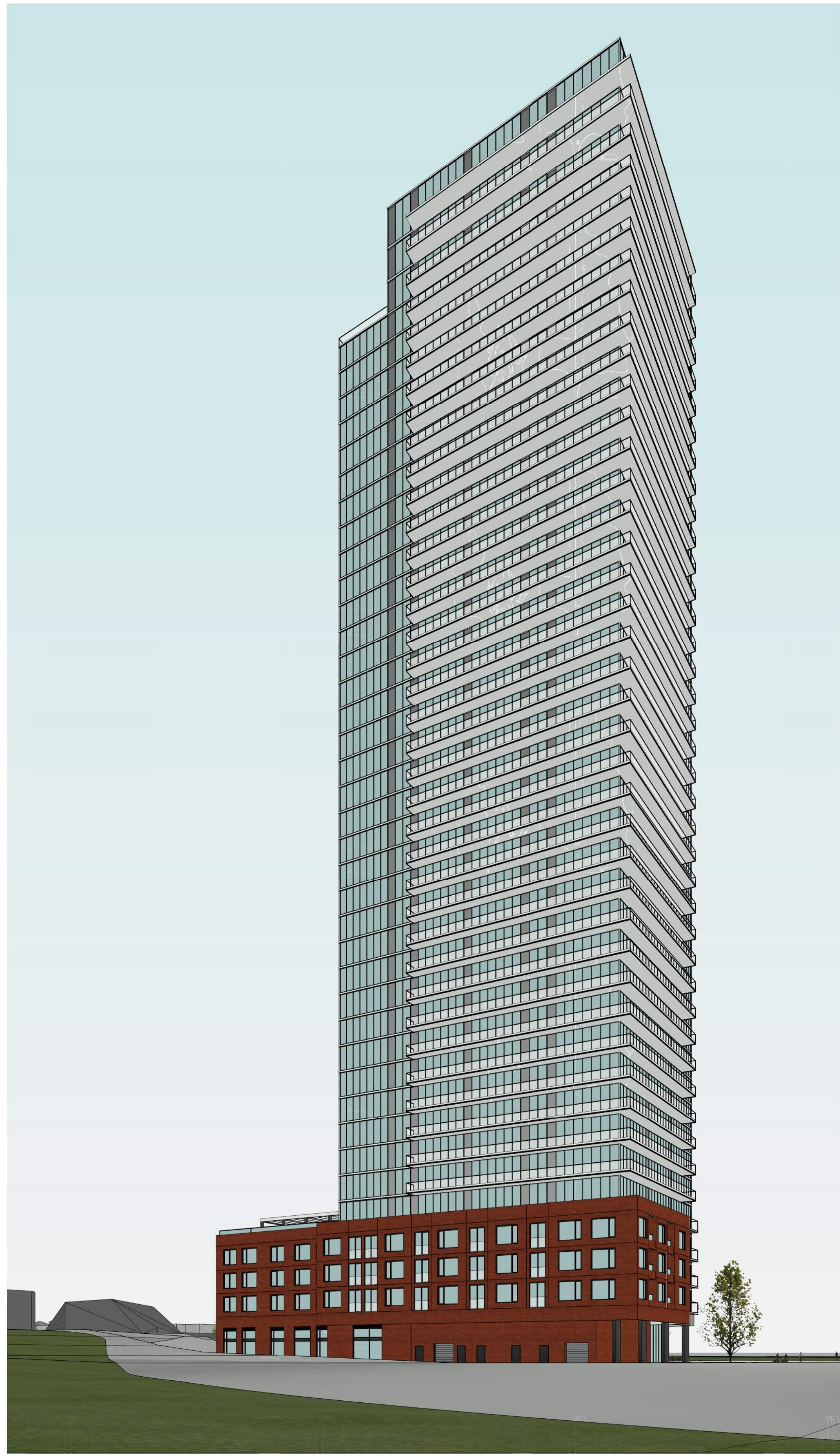
VIEW LOOKING NORTH-EAST
