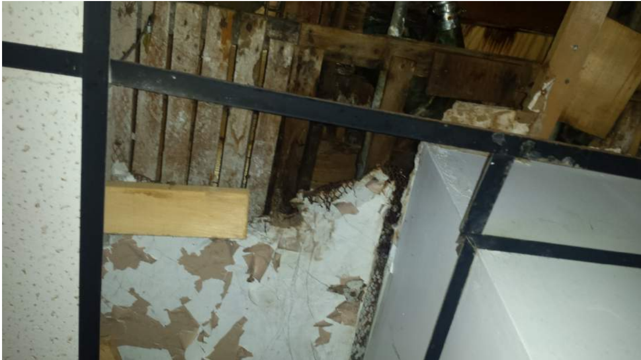
Photograph 5: Exposed ceiling (suspended ceiling tile and plaster lath) at 406 Roosevelt.
