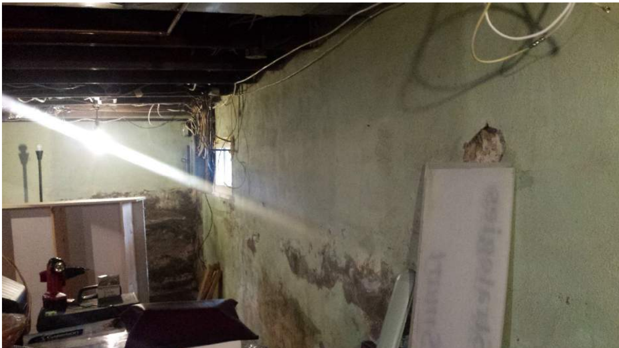
Photograph 6: The basement of 402 Roosevelt Avenue.
