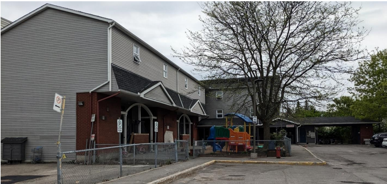
Figure 5: Looking southeast towards Block 4 from the communal drive aisle
