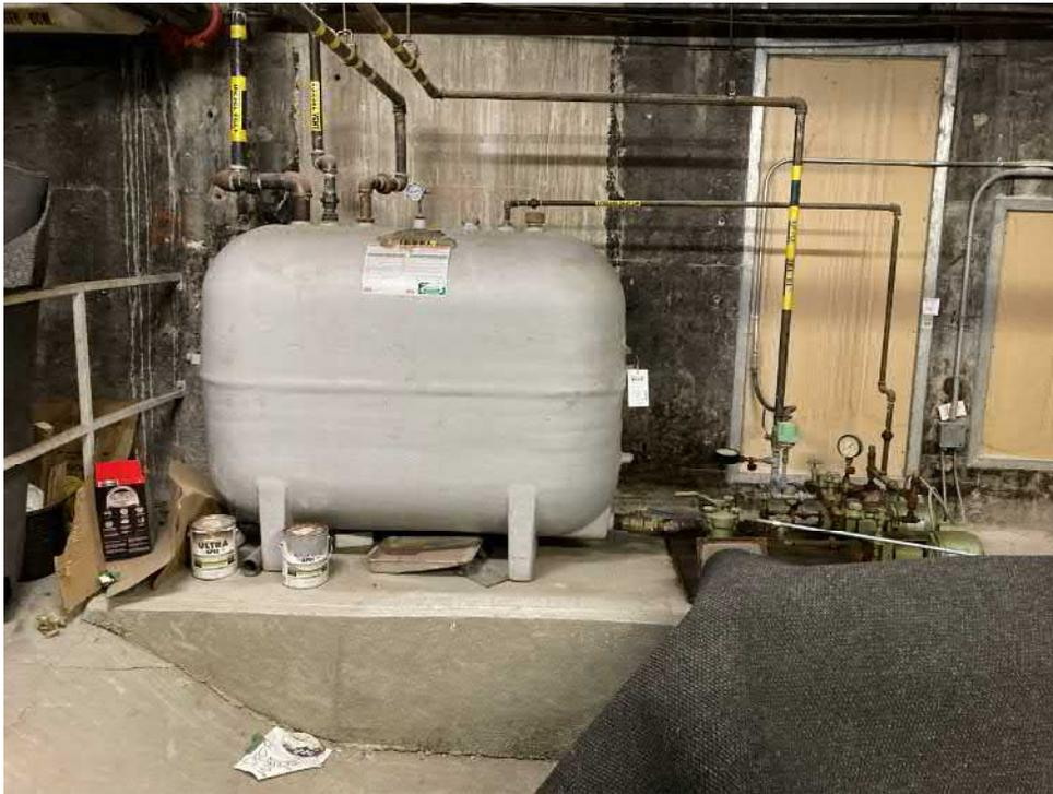
Photo 9: AST containing diesel fuel for backup generator. Tank is in basement mechanical room.
