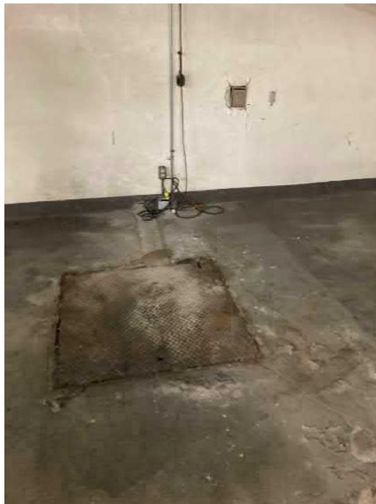
Photo 14: Sump pit in underground parking garage
