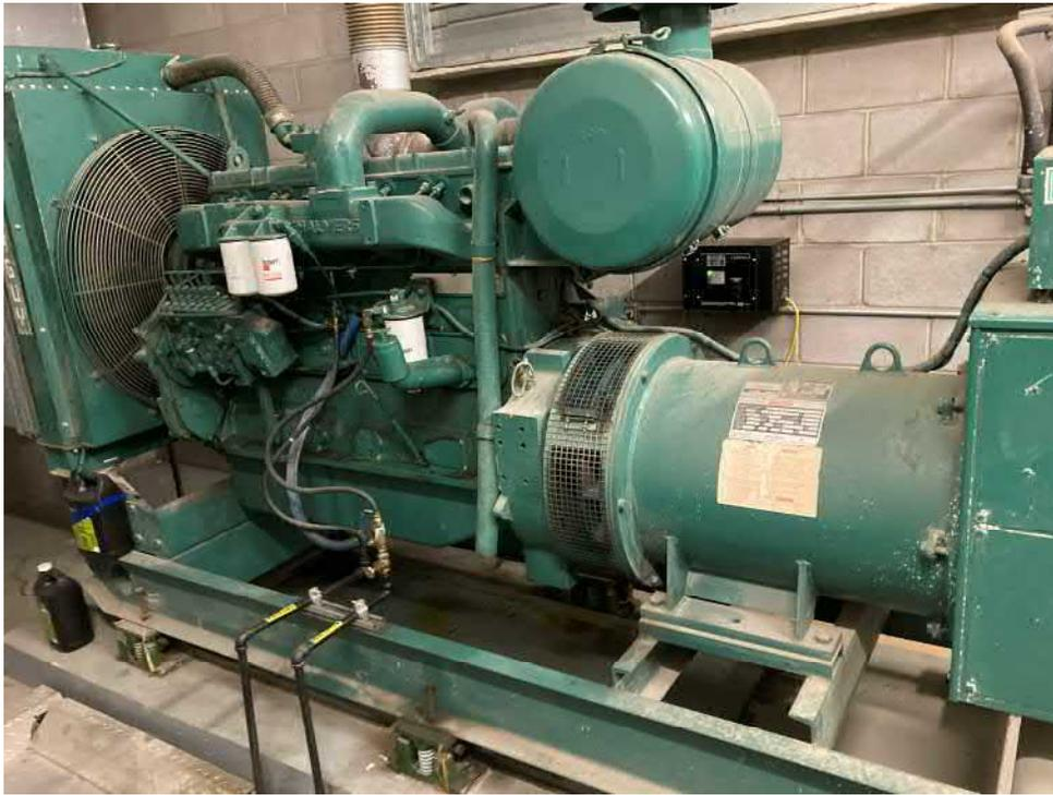
Photo 15: Diesel backup generator in mechanical penthouse (11<sup>th</sup> floor)
