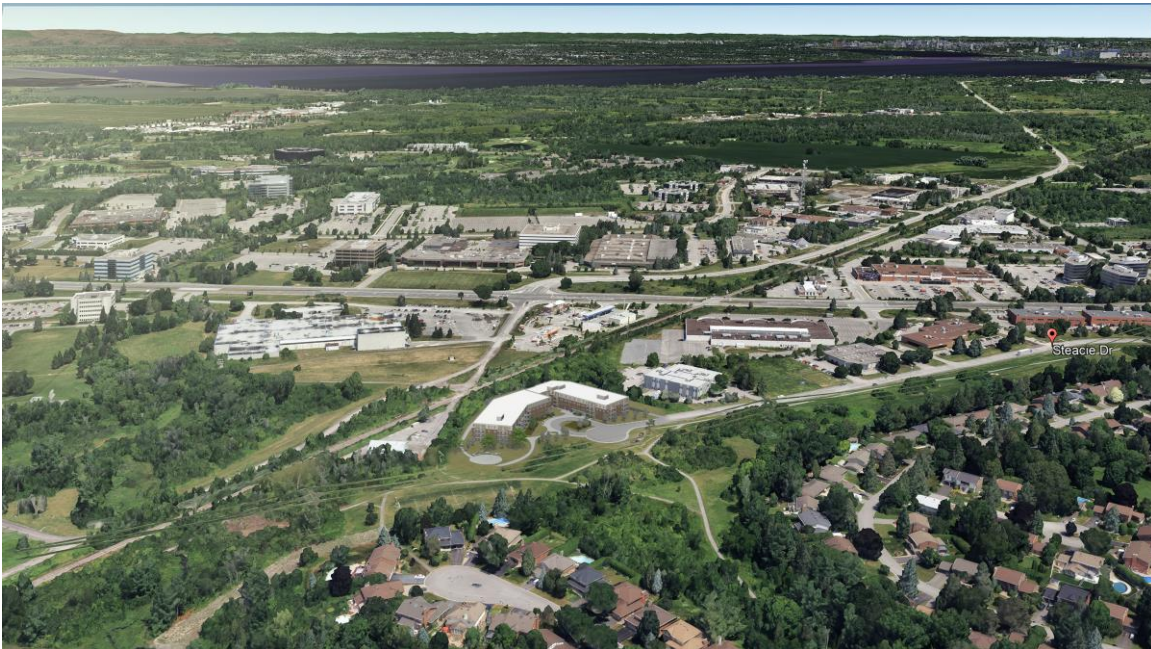
Figure 21: Aerial Image of the proposed development, facing North-East.
