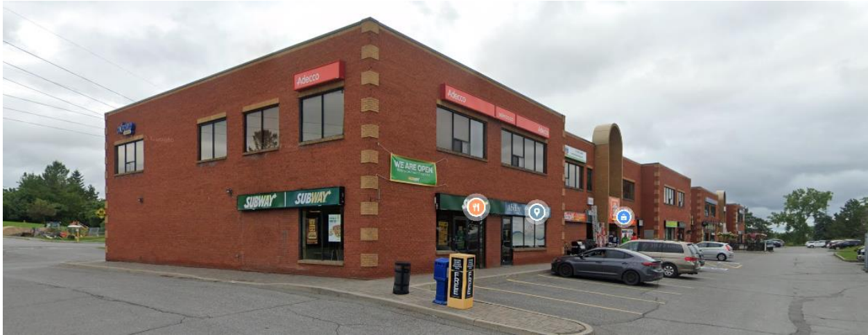
Figure 10: Existing Commercial Plaza, 329 March Road.
