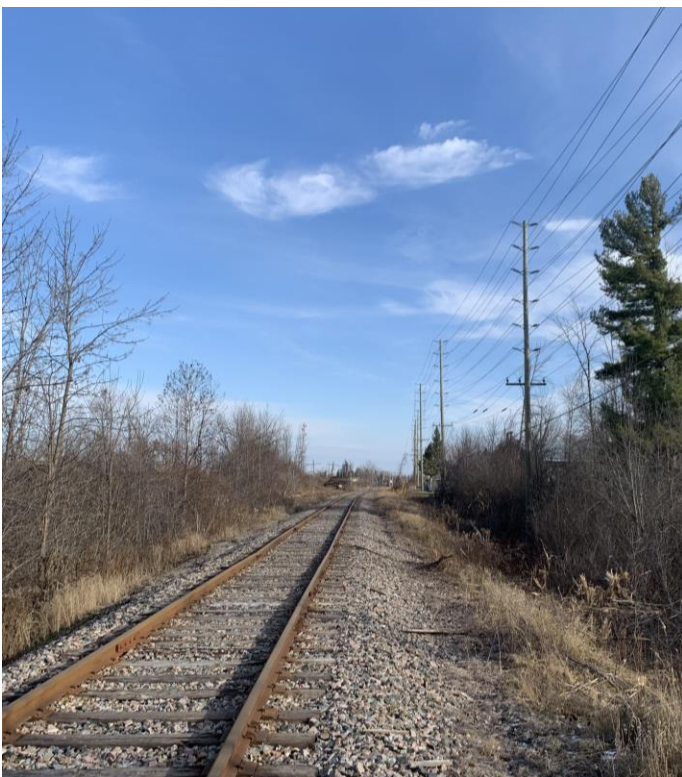
Figure 16: Beachburg/Renfrew Railway Corridor, looking east.
