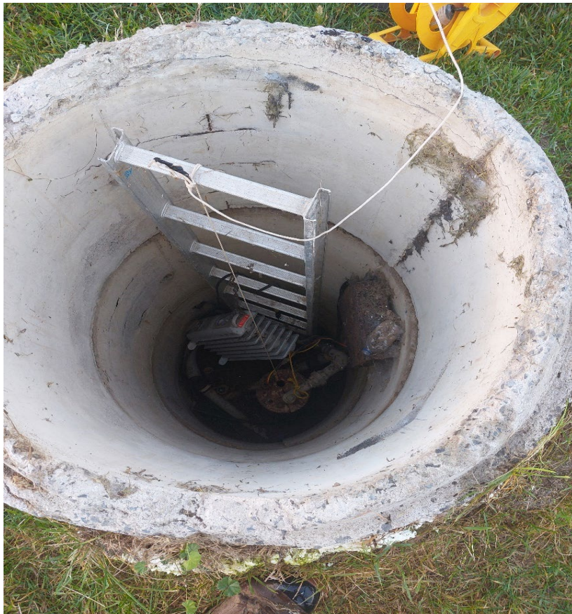
Photo 2 - Interior view of well pit of drilled water well TW-1.
