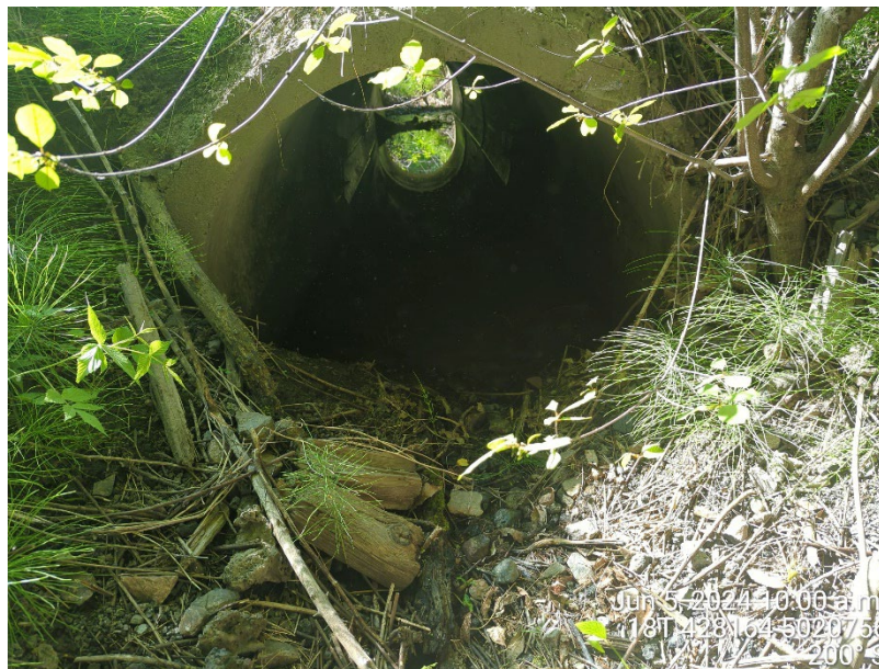
Photo 2: Culvert under the Railroad (June 5, 2024)
