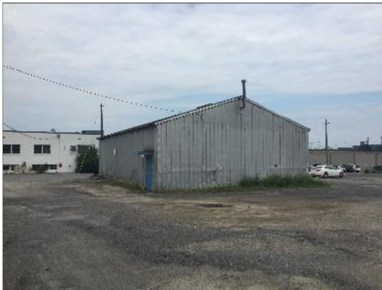
Photo 4 – General view of Site Building D.
