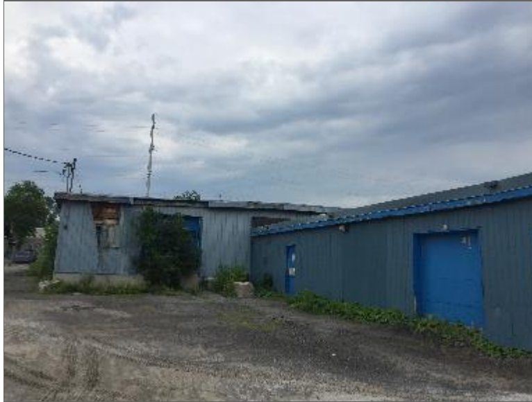
Photo 5 – Site Building E (north elevation).
