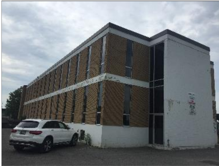
Photo 3 – Site Building C (north and east elevations).
