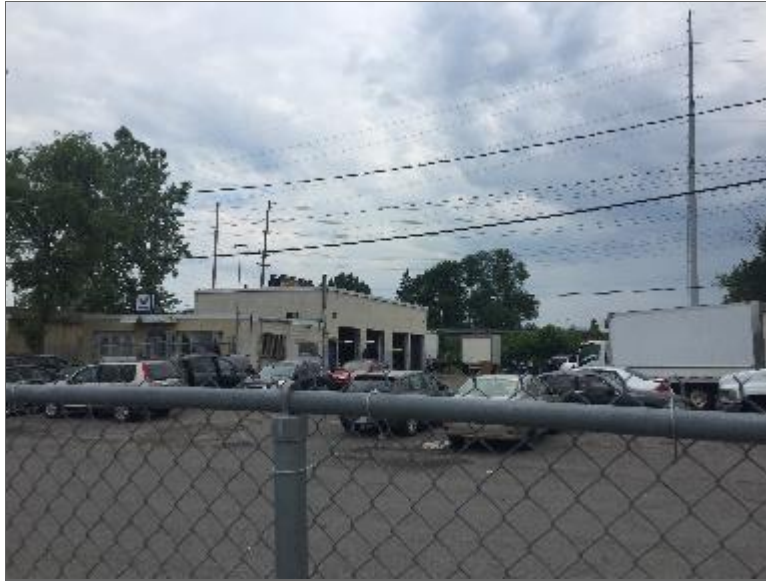
Photo 11 – Property located east of the Phase One Property (i.e., automotive repair/servicing garage (PCA), and property with former PFO (PCA)).
