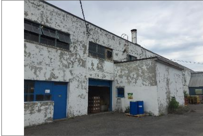
Photo 1 – Site Building A (west elevation).
