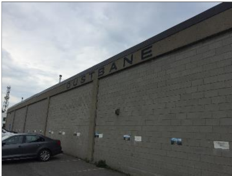
Photo 2 – Site Building B (east elevation).
