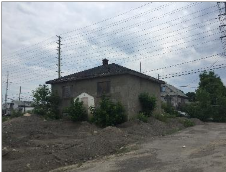
Photo 6 – Site Building F (west elevation).
