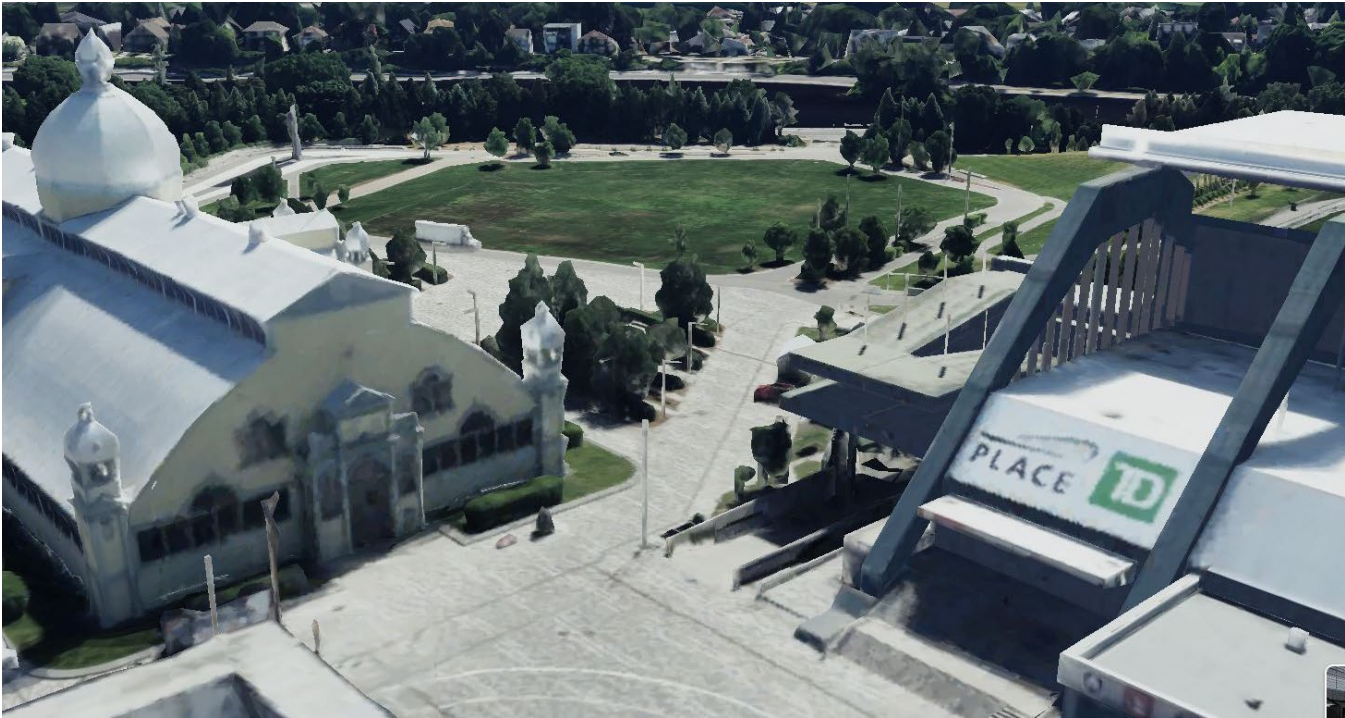
Figure 6. Existing condition looking south-east.
