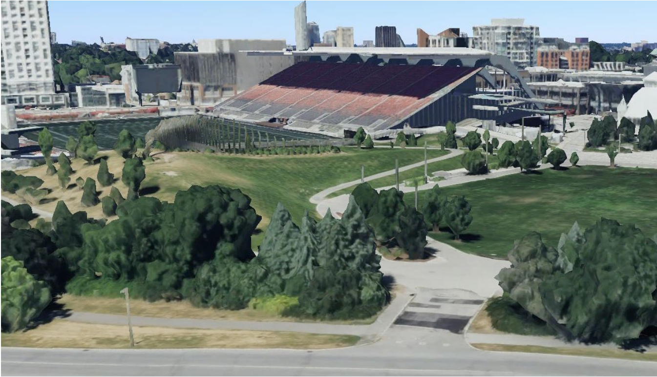
Figure 5. Existing Condition looking north-west.
