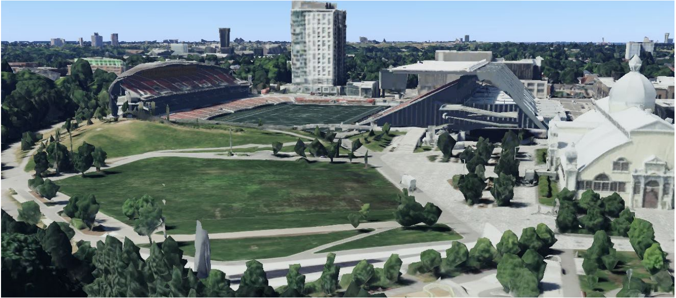
Figure 7. Existing condition looking west.
