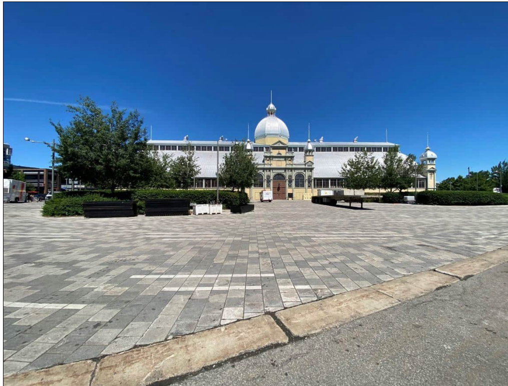
Photo 5: General view of the south elevation of the Great Porch area. Date: 06/28/24 Direction: Northwest
