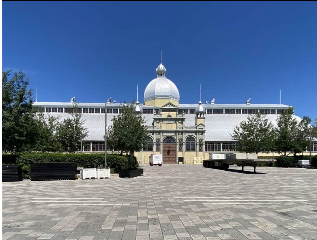
Photo 15: North of Site: General view of the Aberdeen Pavilion. Date: 06/28/24 Direction: Northwest
