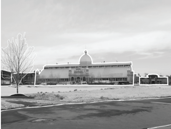
Existing condition of Viewpoint A.
