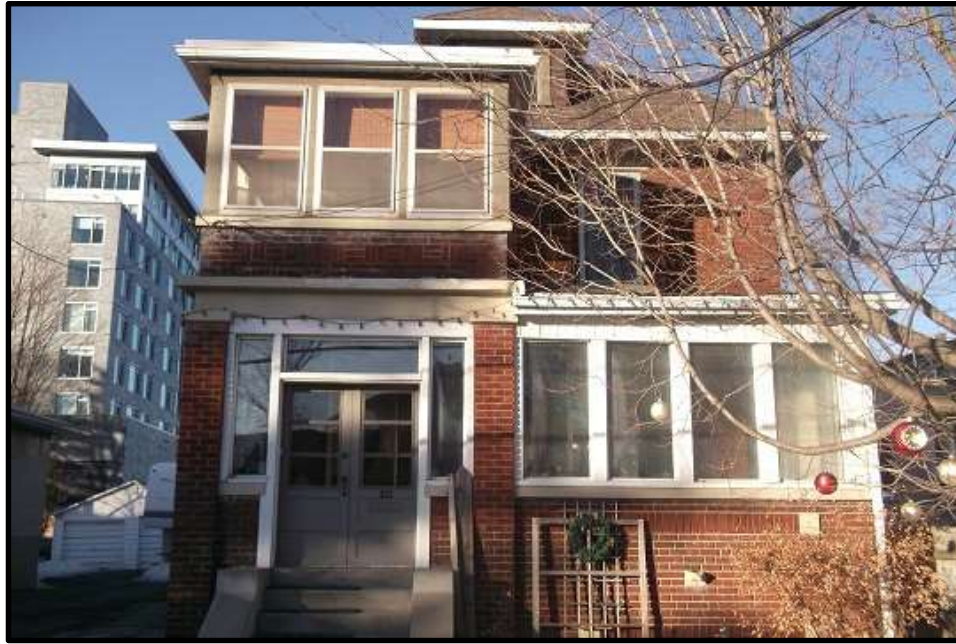
Photograph 3: East face of subject building at 312 Clifton Road, facing west.
