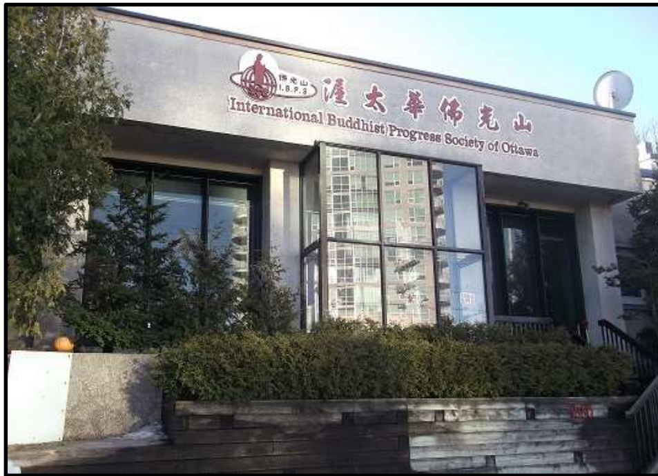
Photograph 1: North face of subject building at 1950 Scott Street, facing southeast.
