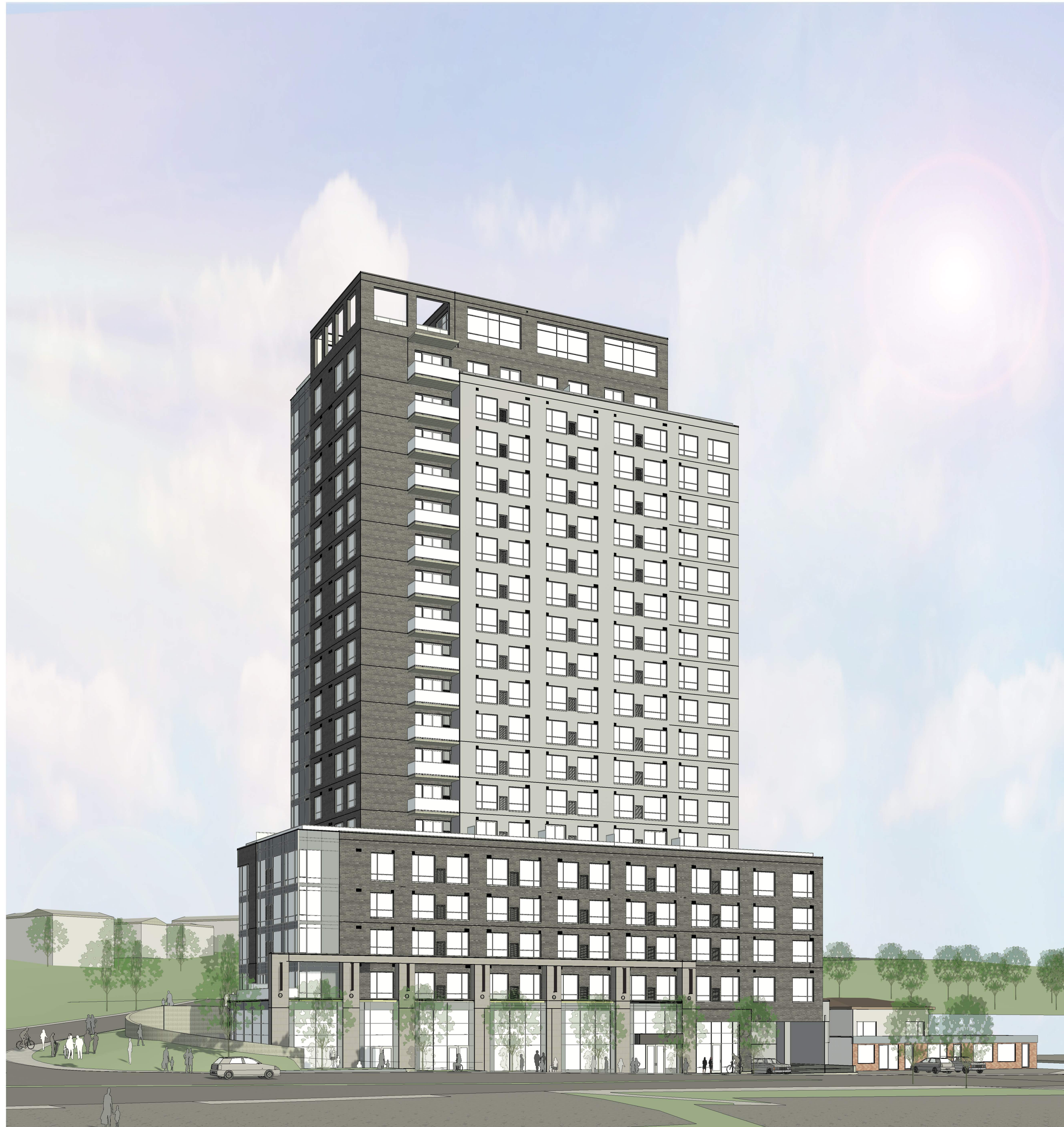
VIEW LOOKING SOUTH FROM ACROSS ST. JOSEPH
