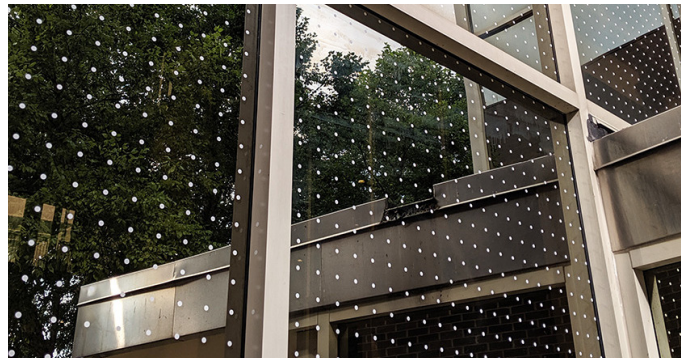
Figure 4.4: Example of Bird-Safe glass using visual markers
