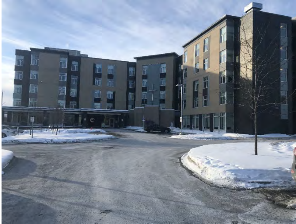
Photograph 1 - The subject property structure facing south from parking lot.
