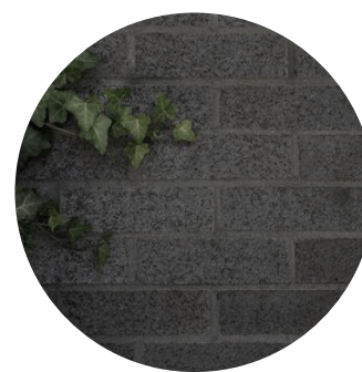
M2 Brick cladding such as "Black Diamond Velour" of Belden or equivalent, "Norman" dimensions.
