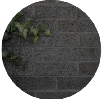
M2 Brick cladding such as "Black Diamond Velour" of Belden or equivalent, "Norman" dimensions.
