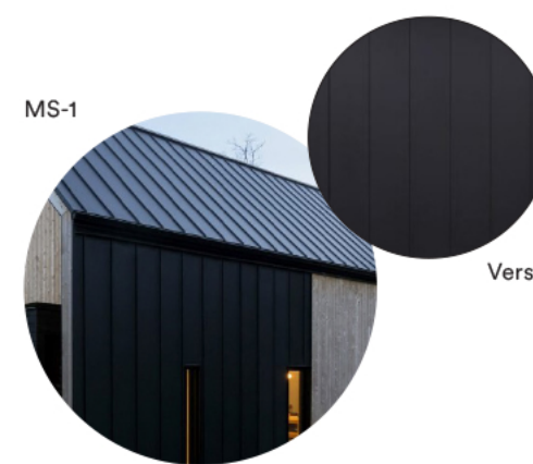
M3 Pinched bead steel cladding such as Mac Metal's MS-1 model when lined on the front and Versa 12" wide panel model in other areas. Titanium black color.
