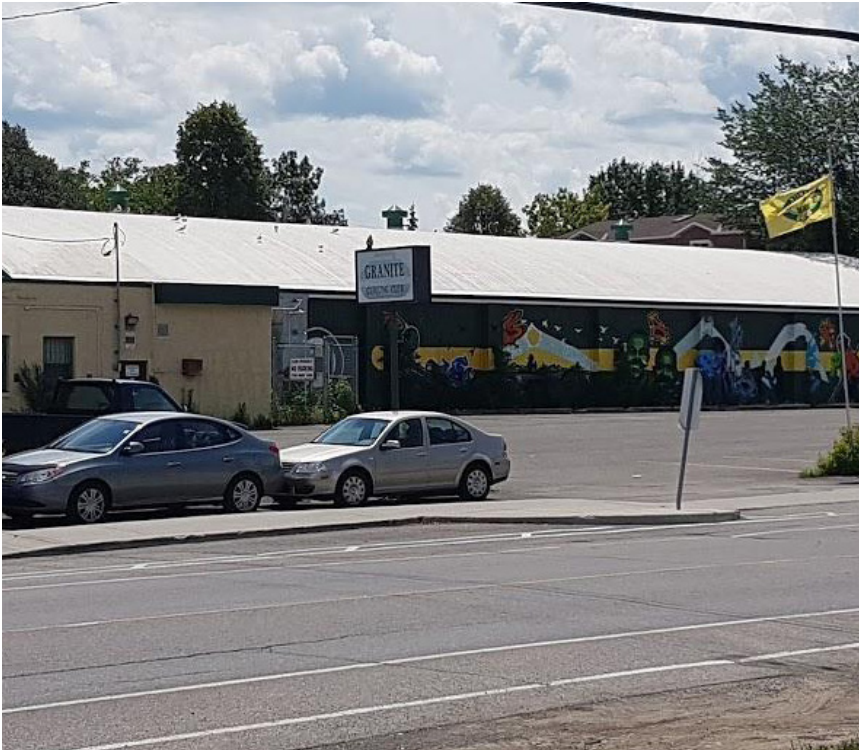
Figure 3.0 - Existing Granite Curling Club, 2026 Scott Street.
