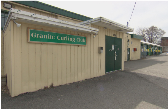
Figure 4.0 - Existing Granite Curling Club, 2026 Scott Street.
