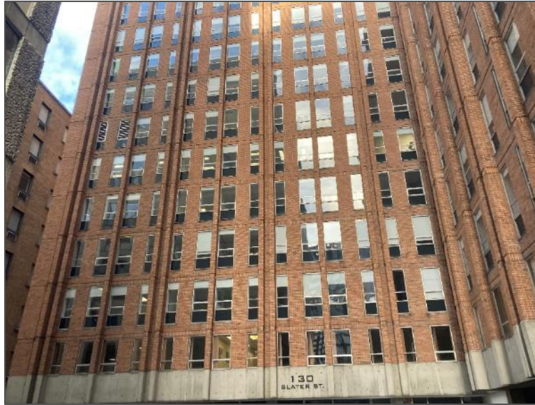
Photo 3 – Southeast elevation of the Site Building.
