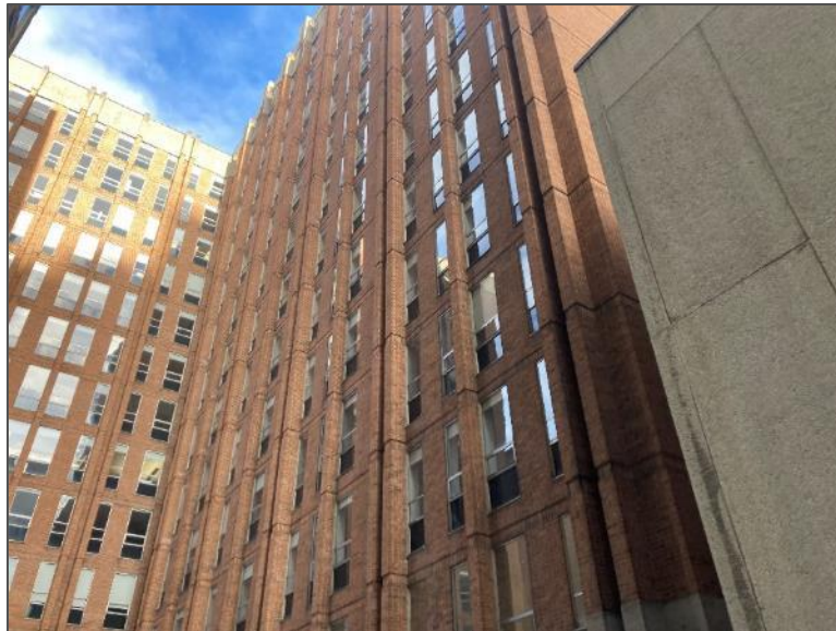
Photo 4 – Southwest elevation of the Site Building.
