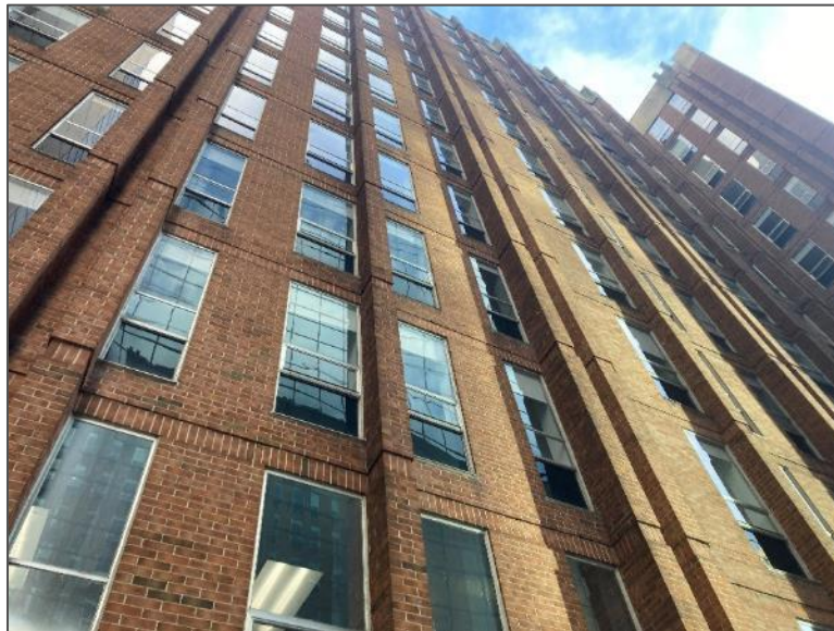
Photo 2 – Northeast elevation of the Site Building.
