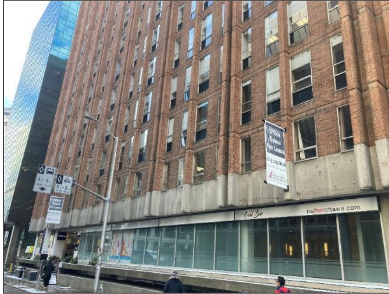
Photo 1 – Northwest elevation of the Site Building.
