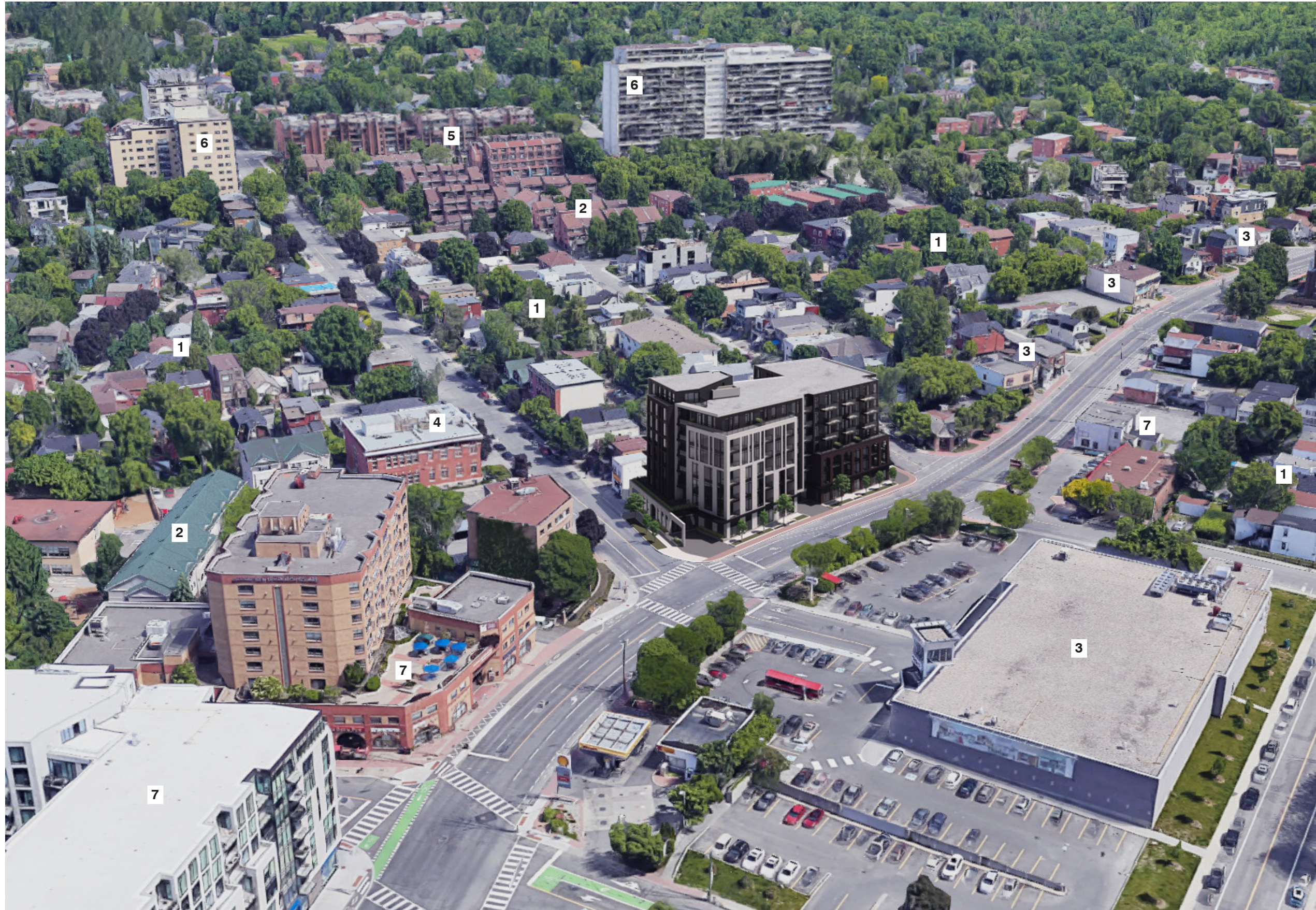
View Looking North
