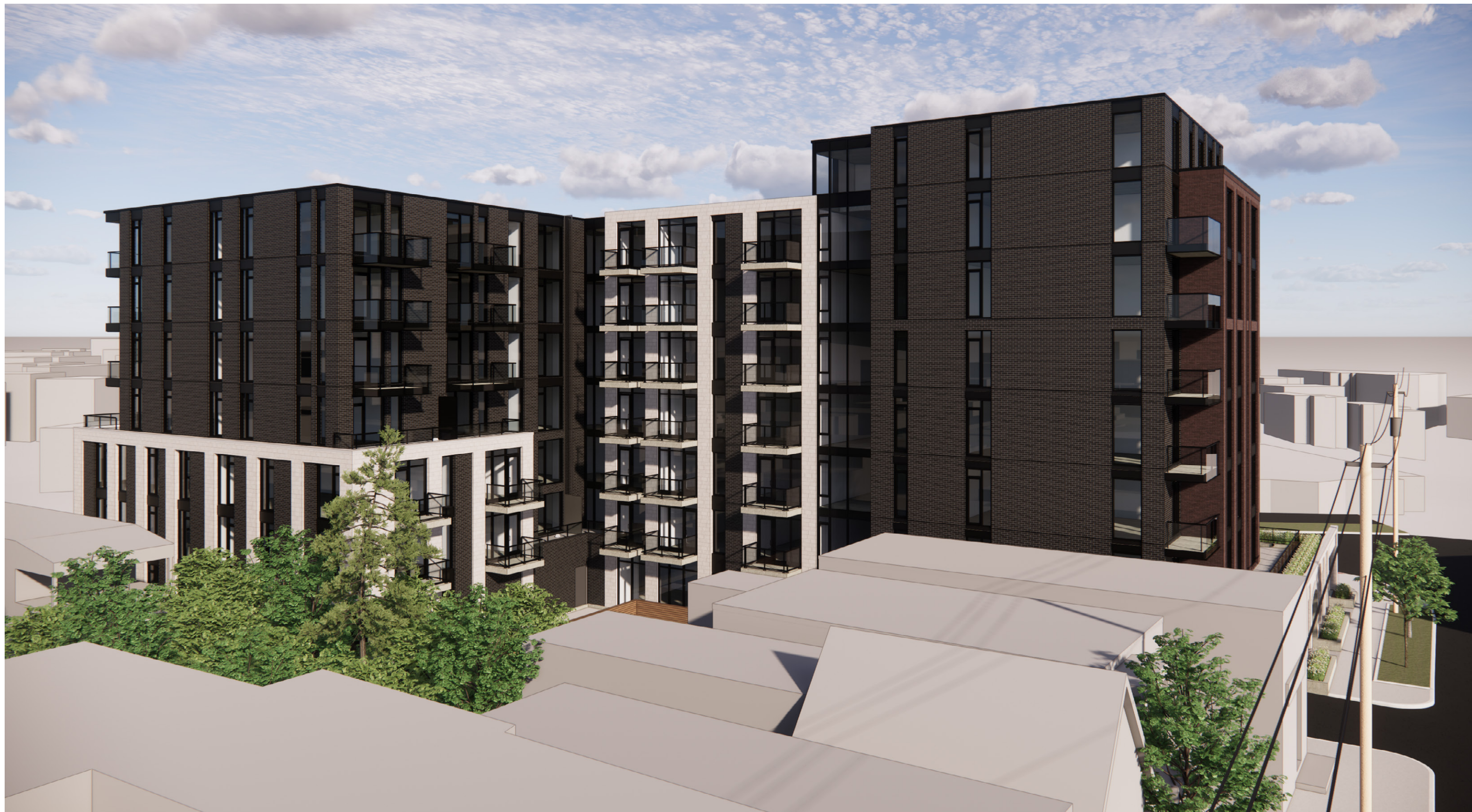
47 BEECHWOOD AVENUE VIEW OF REAR OF BUILDING
