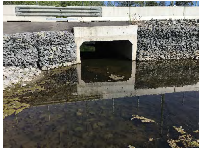
H – Box culvert across Klondike Road, looking northwest
